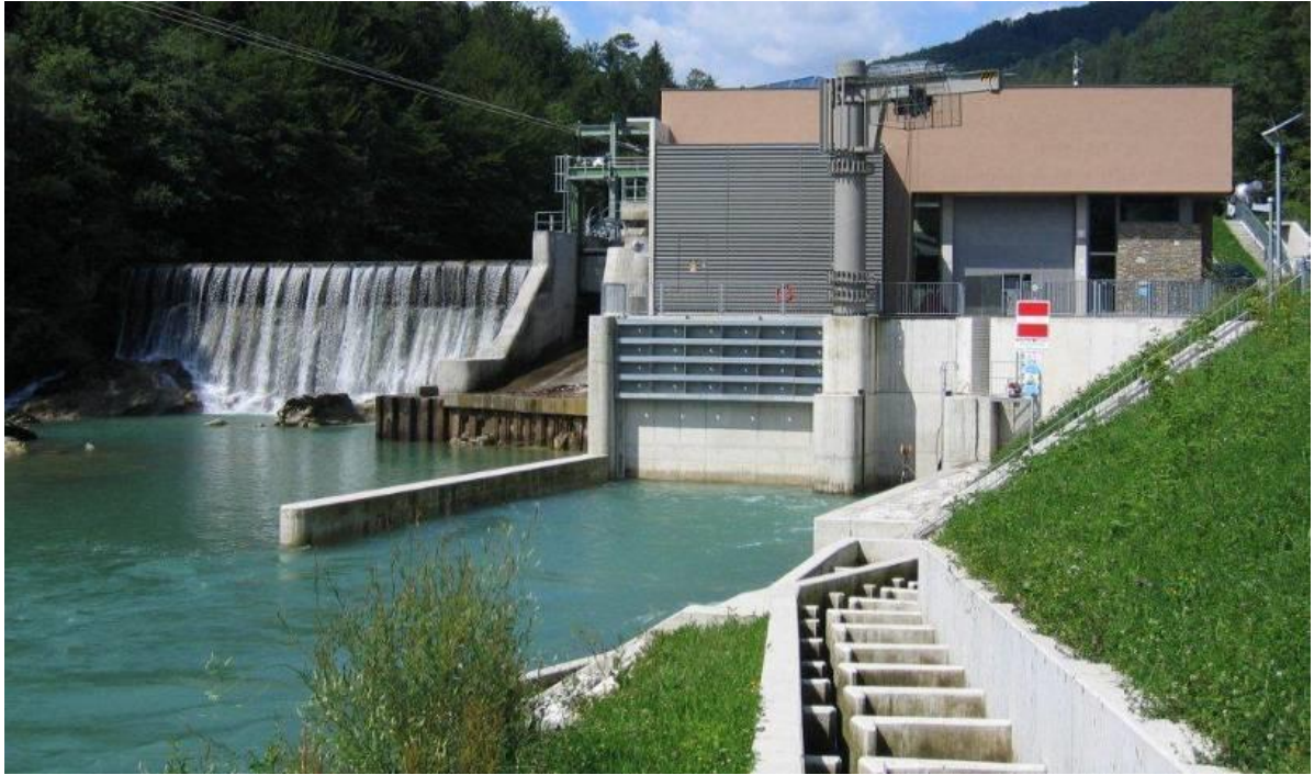
An example of a storage MHE with a cascade fishway
